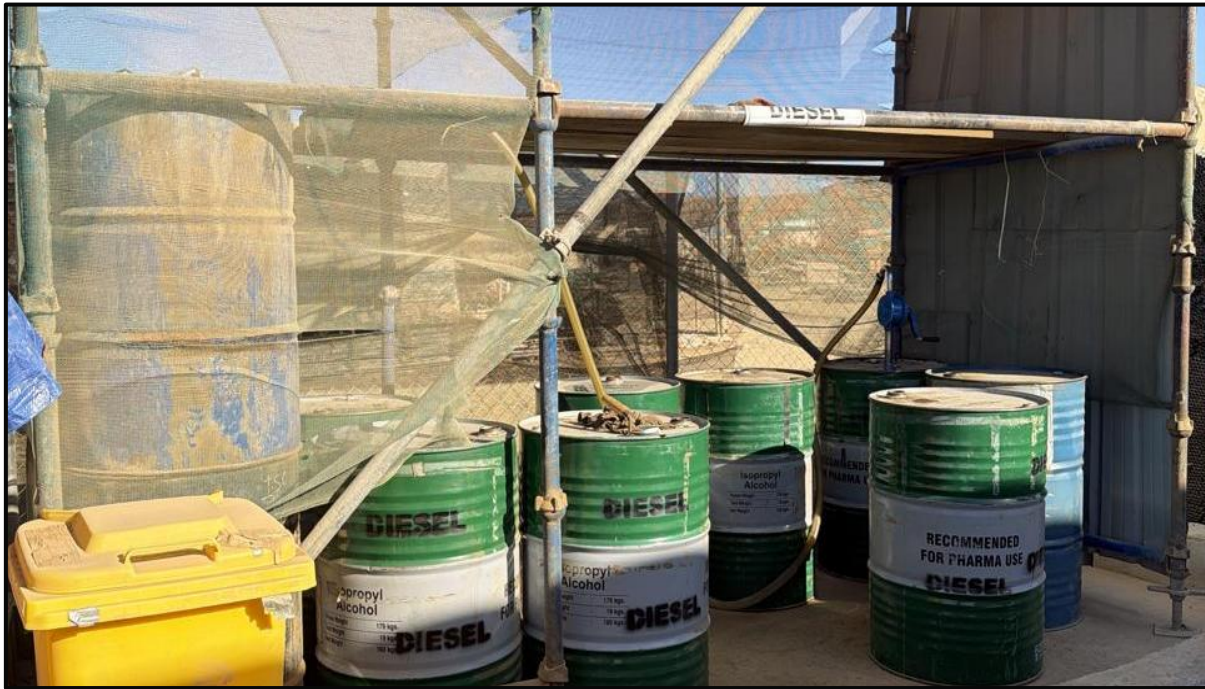
The fuel Storage Area is Bunded, Shaded, covered and away from receptacles.
